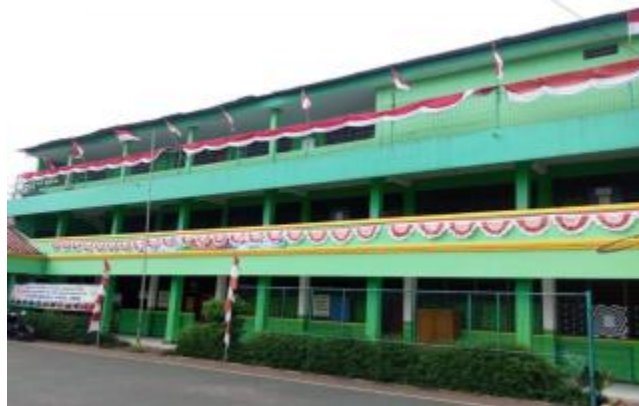
Figure III.1. The School Building of SMP Hidayatul Athfal
